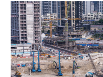
HIGH-RISE BUILDING CONSTRUCTION
