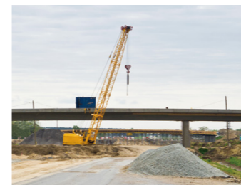
ROAD AND HIGHWAY CONSTRUCTION
